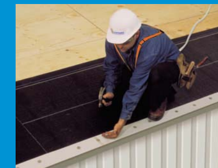
2 Apply base sheet flashing along perimeters and upstands directly onto primed substrate.
