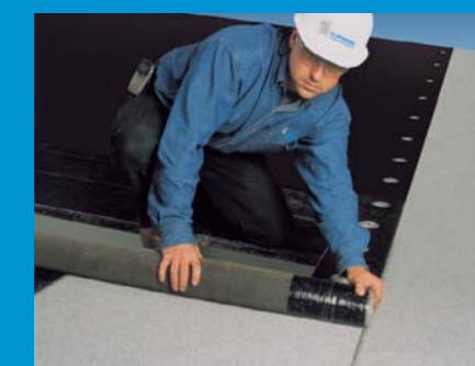
4 Unroll membrane dry onto the substrate at least 20 minutes before installation. Align and re-roll the membrane.
