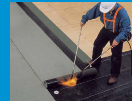
6 Torch (or adhere) Unilay onto reinforcement membrane.
