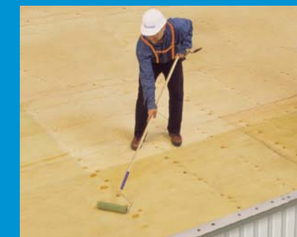
1 Substrates will receive a coat of primer before application of base sheet flashing.
