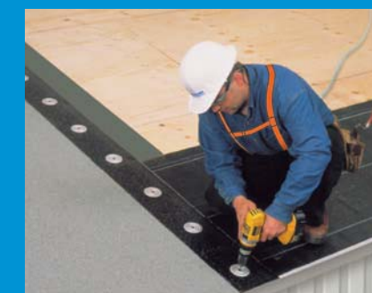
7 Fasten along the edge of the sheet in accordance with Soprema's Specifications Manual.
