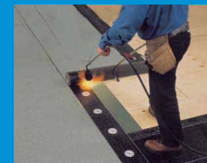
5 Seal joints by heat-welding (or with adhesive).
